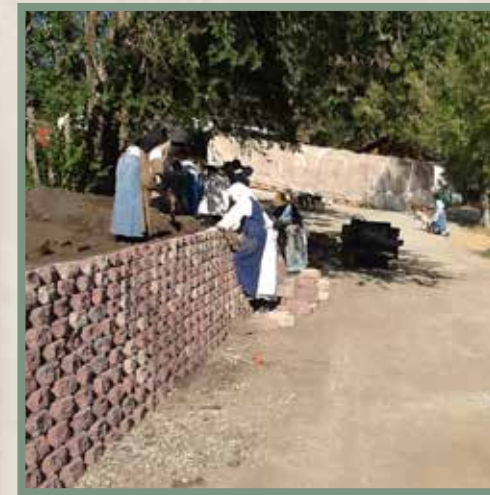
This retaining wall was erected by the new "priest cabin" near the entrance to our Priory.
